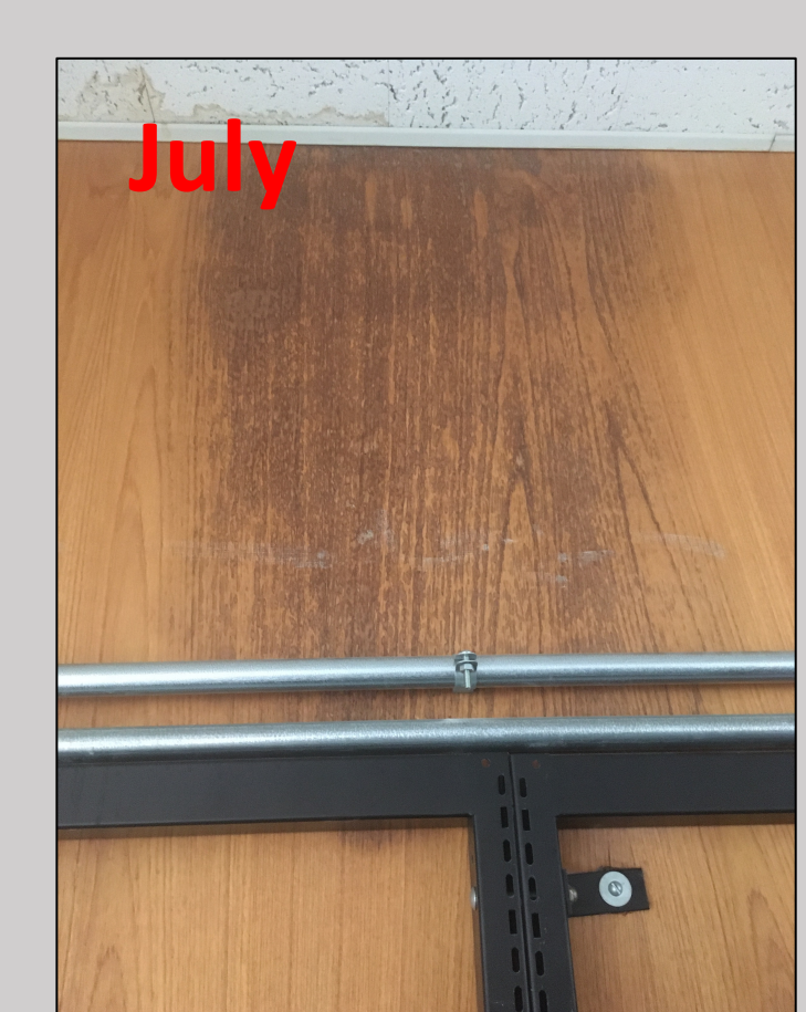
Images documenting change in water staining, demonstrating an active leak.
